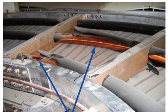
Lubricant residue from an adjacent duct system contributed to LSZH jacket failure.
