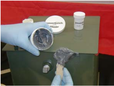
Apply PowerPatch® Sealant over putty patch or leak area
